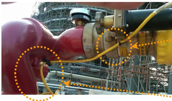
Need Nozzle wire held tight to Monitor between Nozzle and upper cable restraint. Attaching Nozzle wire to the nozzle actuator helps to insure that there are no issues. Alternatively the cable could be routed between the nozzle actuator and nozzle to hold the cable in position.
