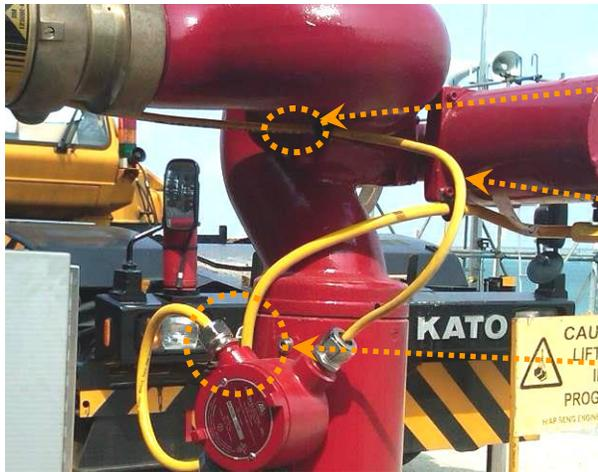
Need Nozzle wire held tight to Monitor between Nozzle and upper cable restraint.
